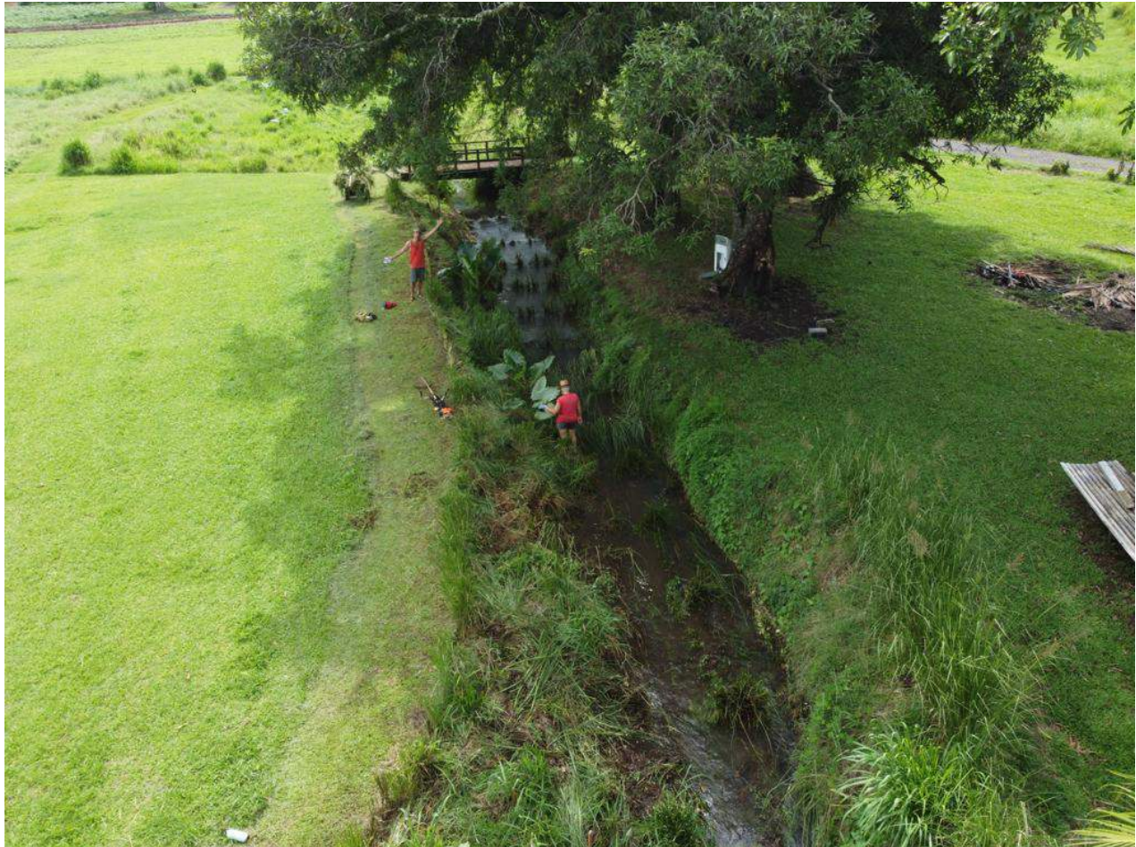
Figure 5. Aerial photo of Vetiver plantings on the shaded section of the 120m planting site. 17/3/23
